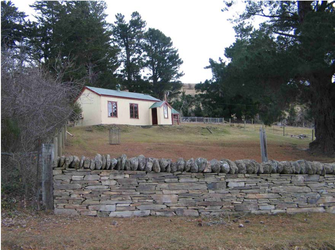
Figure 8: Church of St. Alban the Martyr, north elevation and setting
